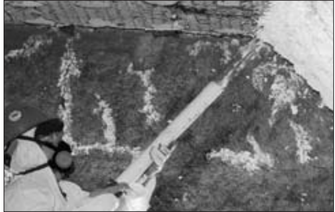
Foamfrax Installation
