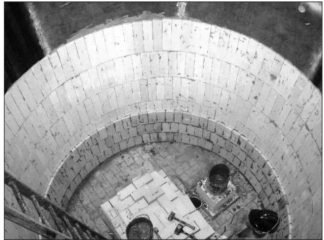
Safety lining brick installed over Silplate 1308.
