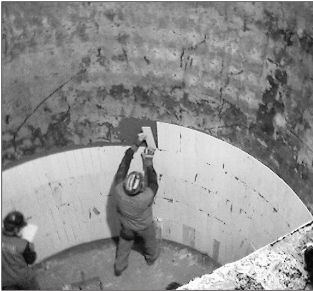
Silplate 1308 installation in a steel transport ladle.
