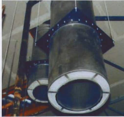
Prefabricated fire resistive duct enclosure system
