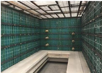
*Photo-1 Casing during stud welding*
