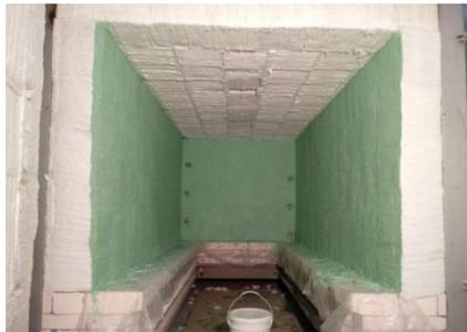
*Photo-4 Lining after application of Silplate Mass S*
