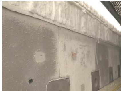
Photo-4 Refractory lining to the base of the walls
