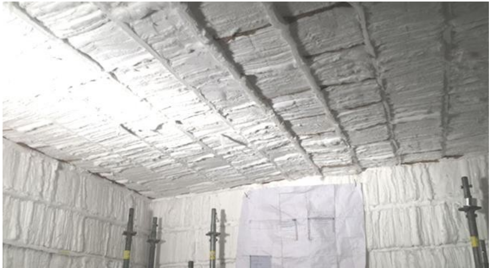
Photo-3 Module lining on the roof and walls before tamping
