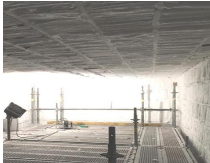
Photo-5 Lining during the installation
