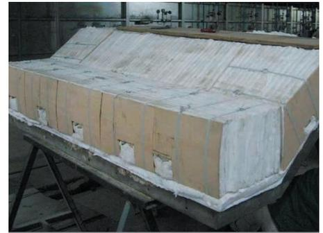
*Roof section during installation, prior to lifting onto the kiln roof*
