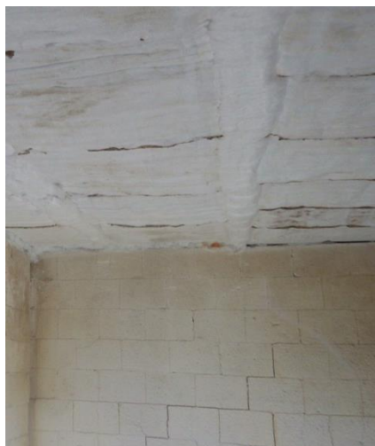
Photo-5 Roof lining
