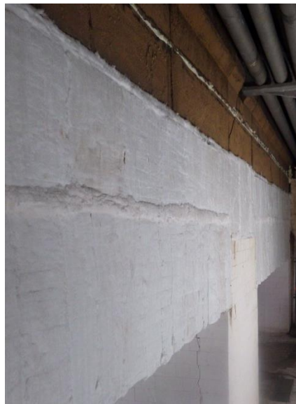
Photo-4 Corner lining
