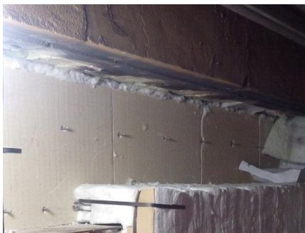
Photo-2 Isofrax 120LD Board back-up layer
