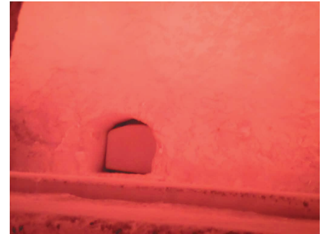
Internal view—no loss of Silplate Mass 1500 since December 2014
