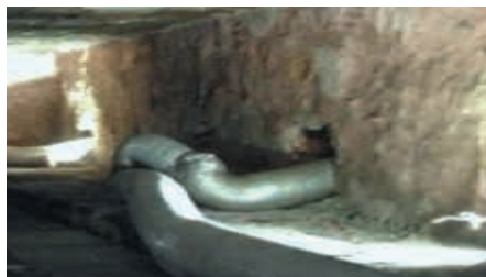
Furnace walls after installation
