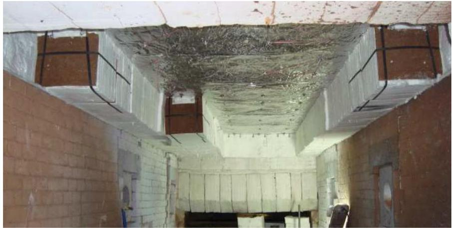
Photo-3 Modules during installation of the arch section
