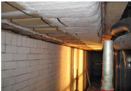
Photo-4 Custom fabricated corner modules
