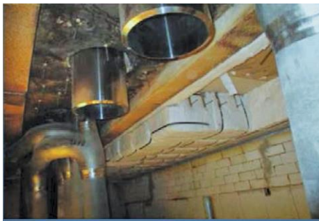
Photo-1 Arch modules being installed
