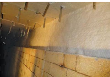
Photo-3 Back-up blanket utilized behind modules
