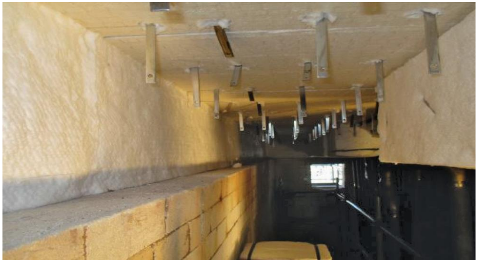
Photo-2 Various anchoring types may be utilized
