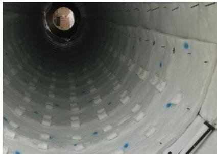
Photo-4 Isofrax Blanket patches applied over the fixing washers
