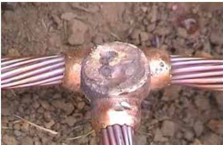
Photo-1 Exothermic welds have high mechanical strength and excellent corrosion resistance due to the purity of the metal produced in the process.
