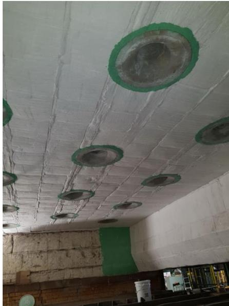
Photo-3 Lining after installation
