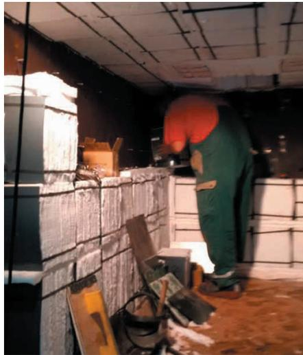
*Furnace side and end wall lining during installation of 200mm thick modules.*
