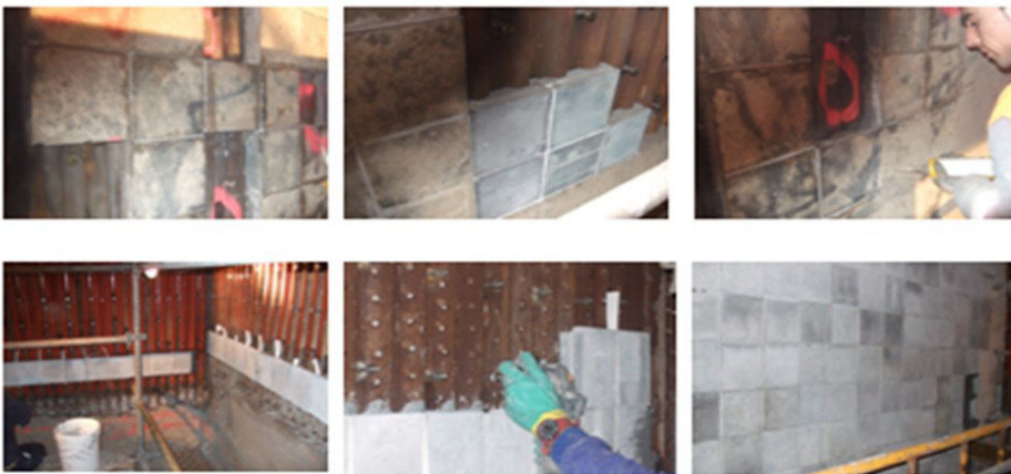
Typical Incinerator Lining Repair & First Lining
