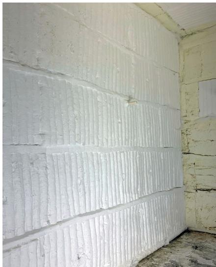
Photo-3 Kiln lining - wall installation
